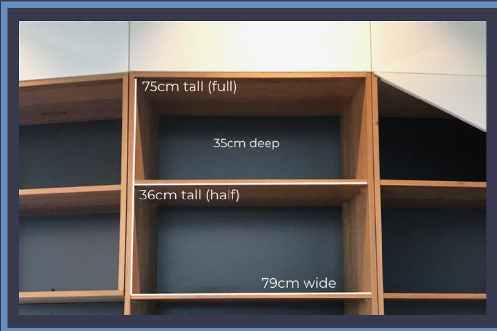
There are 6 square "full" sized boxes that can be adapted to rectangular "half" size by installing a shelf (see left). There are also 6 "half" sized boxes that are not changeable.
